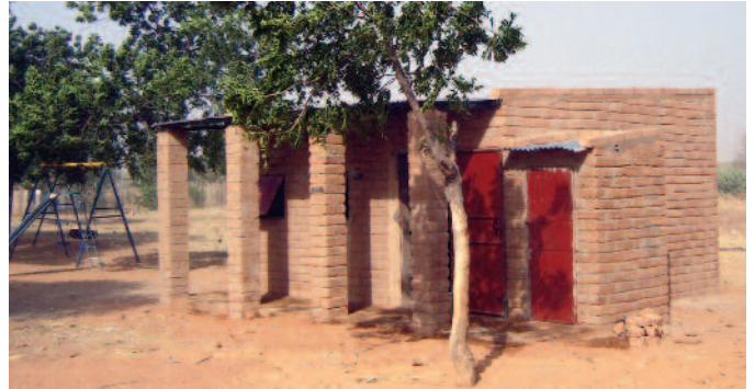
The new pre-school classroom building at Dogon Gao with external closet.
